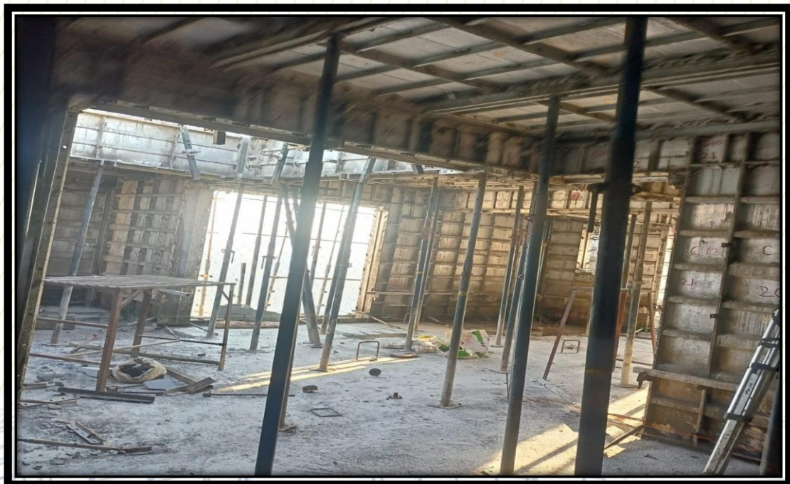
VISIT TO ALU FORMWORK CONSTRUCTION BUILDING HINGEWADI PUNE
